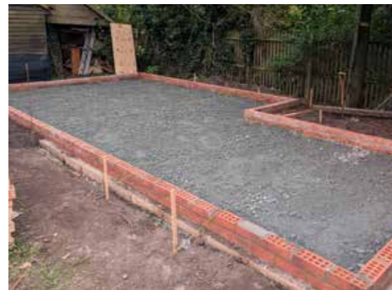
After a lot of hard work, the base was finally ready.
