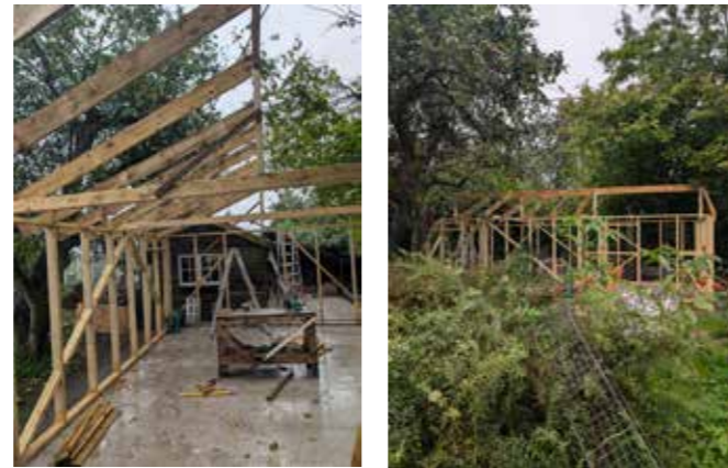
The walls went up and the roof went on fairly easily.
