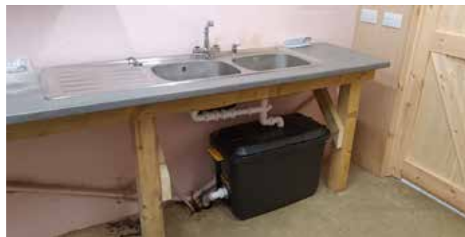
Clay trap under the sink
