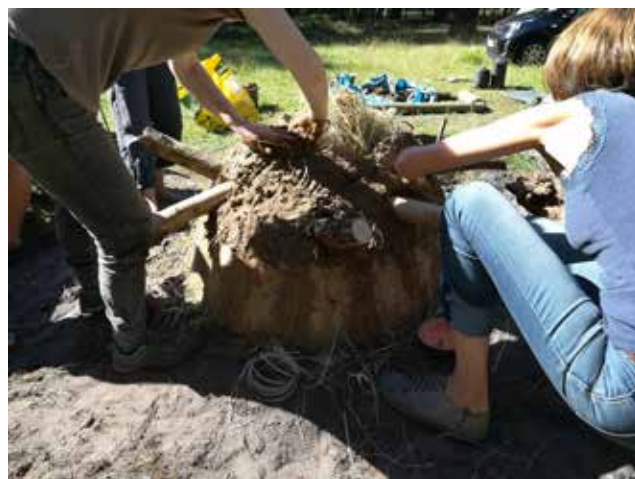
Building the dome on top of hay
