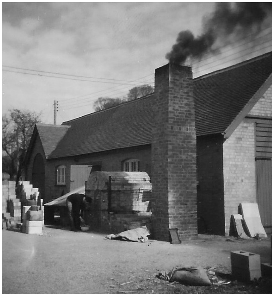
Building the kiln at Avoncroft Pottery, Hampton Lovett, 1955
