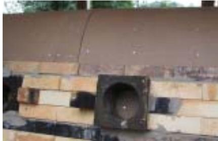
Stoking hole in arch wall
